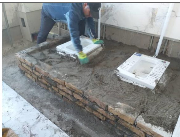
Photo 6: Installation sanitary units, March 2024
