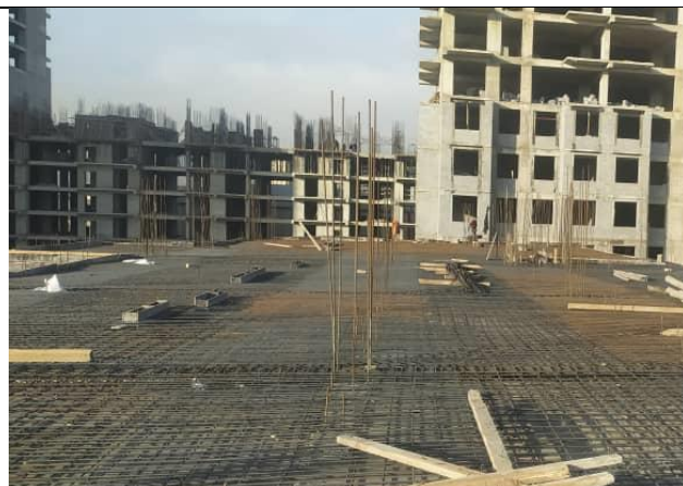
Photo 14: Floor reinforcement, April 2024
